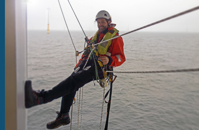
Wind turbine repair worker rappelling on site.
