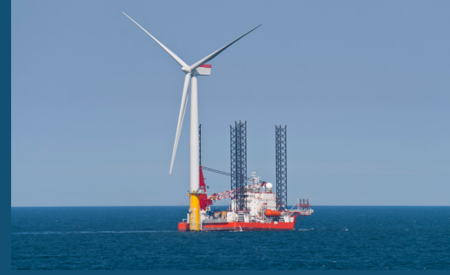
A jackup rig vessel constructing an offshore wind turbine.
